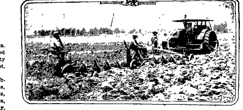
45-h. p. Traction plow in operation. This picture shows our 45-horsepower traction plow sowing raw land, 25 to 30 acres per day, at an expense of less than 50c an acre. plows a strip 16 feet wide at one operation. This is just one item of the big saving on our plantation. This outfit does the work of ten teams.
