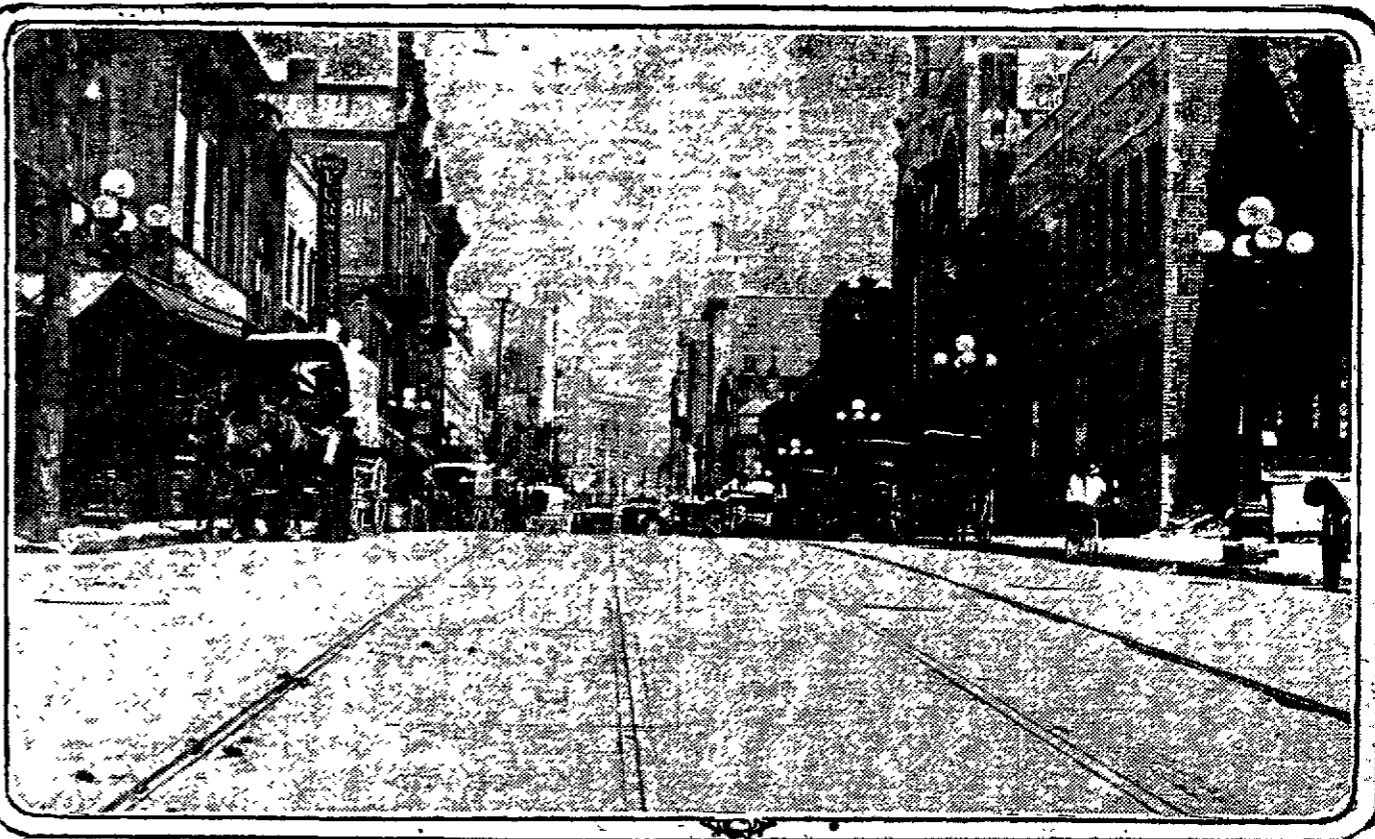
Photo by Francis E. Price, Staff Photographer. Scene showing Whitehall street, looking north from a point between Garnett street and Trinity avenue. The steep grade is being removed. At this point a cut of eight feet will be made and the dirt will be used for the grade.
