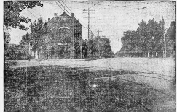
Intersection of Hill Street and Prince Avenue, Athens, Ga. 20,500 square yards of two-course concrete pavement, seven inches thick.
