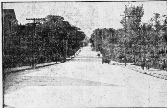
Walnut Street, Macon, Ga., Carries Heavy Traffic from Adjoining Counties, 46 feet wide; eight inches thick; laid three years ago and in perfect condition.
