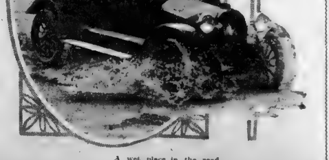
A wet place in the road.
